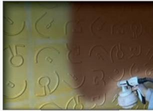
After the drying time of the special-primer (about 60 minutes), the 3D panels can be painted as desired. Common variants are wall paint, latex paint or varnish.
