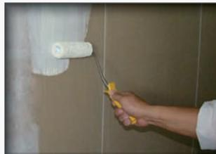
Divide the surface where the 3D panels are going to be glued on. Apply the special-glue to the surface (wall/ceiling) and also on the back of the 3D panels with the help of a roller. Don't miss any gap or edge.
